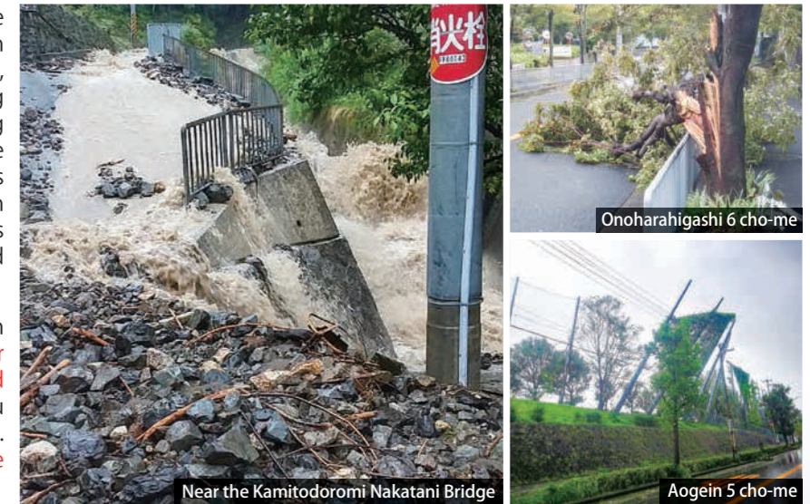
Near the Kamitodoromi Nakatani Bridge
